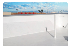
Parapet and wall flashings
